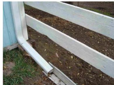
Figure 2. Shed with gutter drainage system. Gutters prevent roof drainage from entering lot.
