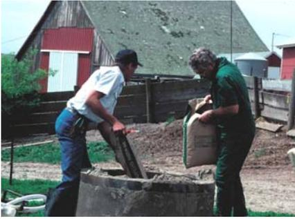
Figure 5. Sealing an unused well.
