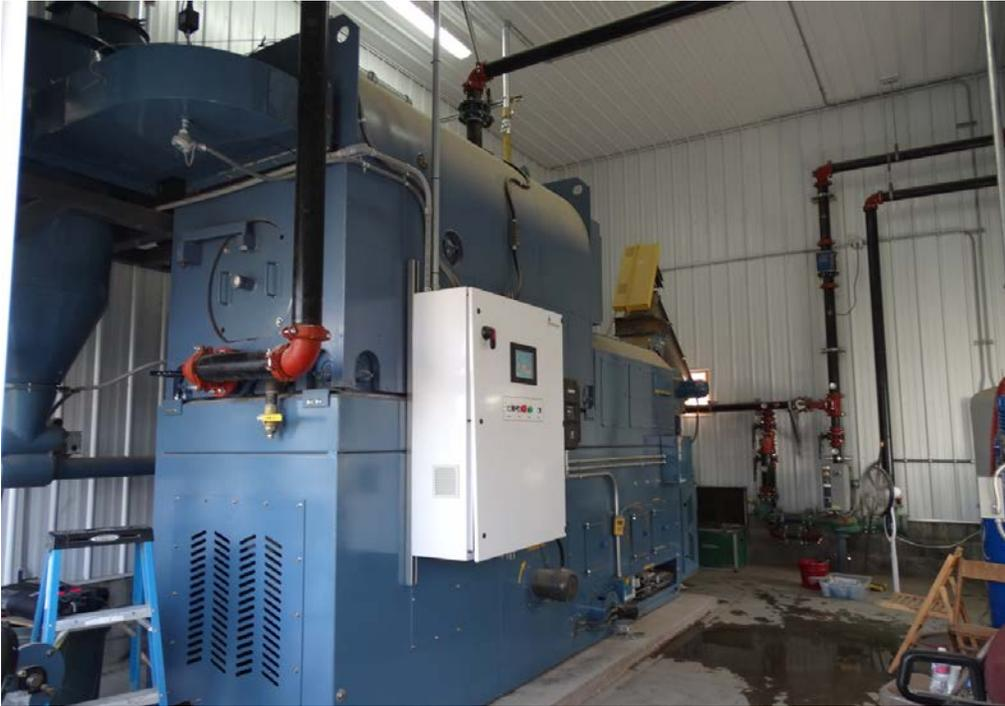
**Figure 3.** Blue Flame stoker and boiler. The boiler sits on top of the combustion system.
