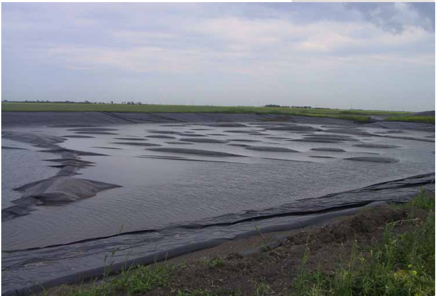
Figure 3. Impermeable manure storage covers require additional management to handle precipitation or debris that may accumulate on top of the cover.
