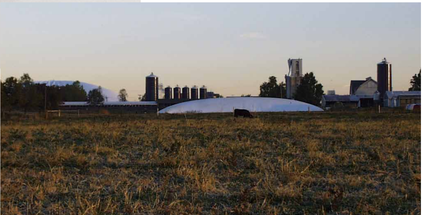
Figure 2. A positive air pressure manure storage cover (Source: Ted Funk, University of Illinois)
