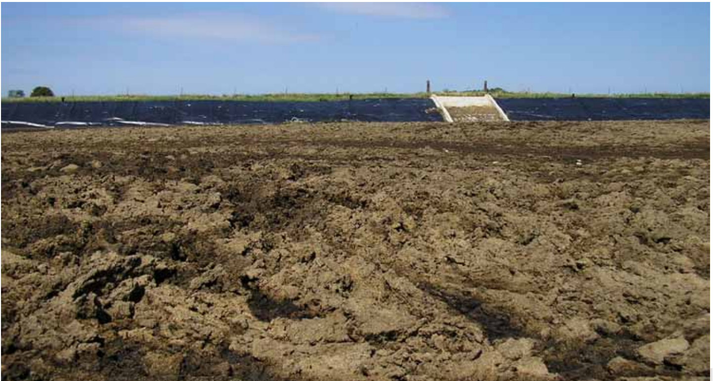
Figure 1. A natural permeable crust on a lined dairy manure storage facility (Source: Kevin Janni, University of Minnesota)
