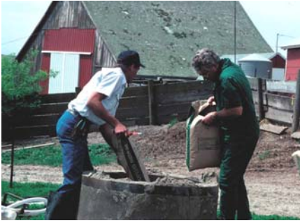
Figure 5. Sealing an unused well.
