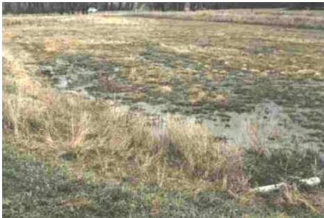
Figure 4. Vegetative filter using gated pipe to take runoff from a lot to a brome filter.
