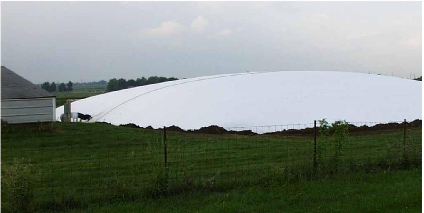
*Figure 1. Positive air pressure covers are filled with air from a blower.
