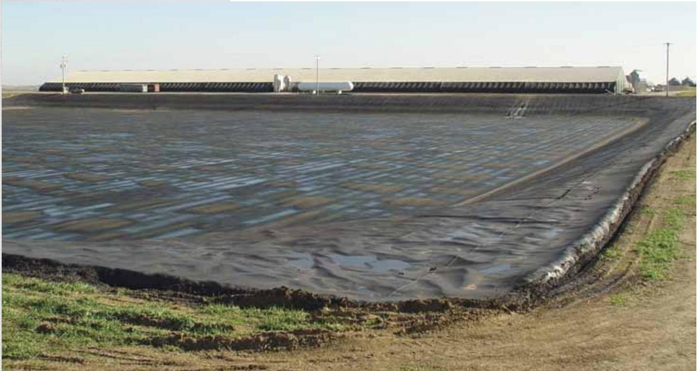
*Figure 4. This floating impermeable cover was installed over an existing earthen manure storage lagoon.*
