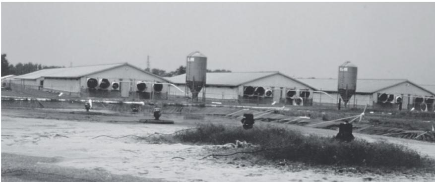
Figure 43-8. Aerated lagoons treating flushed swine manure.
